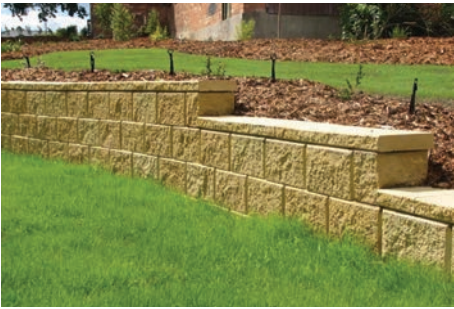
Stepping down using a half corner
